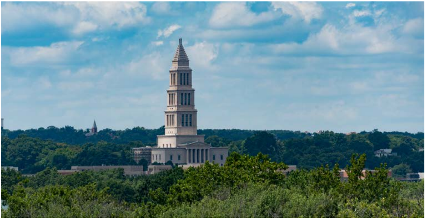
Inspiring as ever, the Memorial's tower now shines more clearly as the exterior restoration nears completion, as the scaffolding moves to the rear portion of the building.
