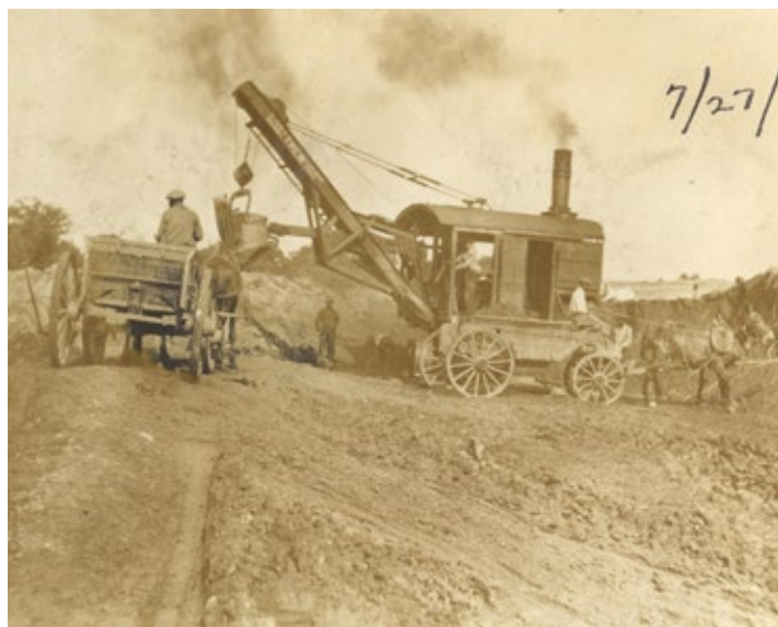
Men at work with steam shovels and mules during the excavation and landscaping of Shuters Hill, July 27, 1922.
