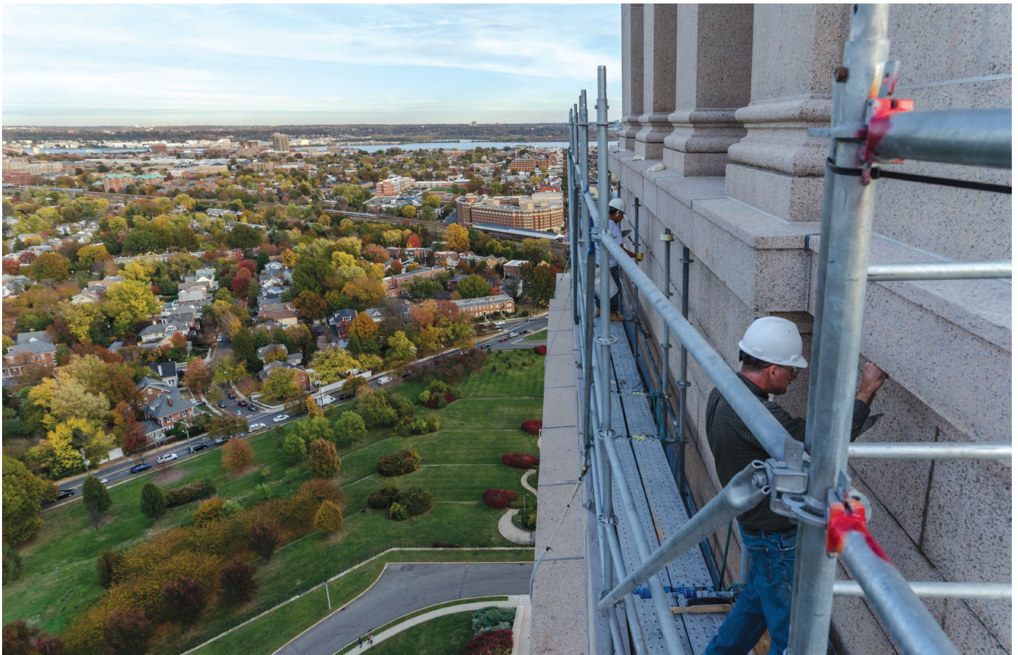
Workers busy re-pointing (replacing mortar) on the exterior of the Memorial's seventh and eighth floors, November 8, 2016, with Old Town Alexandria in the background.
