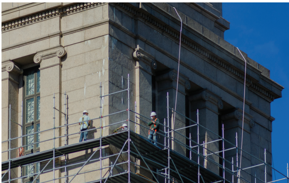
The Memorial's stonemasons at work removing degraded mortar from the southeast corner of the sixth floor.
