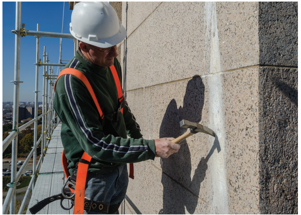
Paul Keegan, the master stonemason in charge of the exterior restoration work, demonstrates the removal of calcium nitrate deposits on the exterior of the Memorial's sixth floor. These unsightly mineral deposits are formed by salts leached out of the stone by rainwater and stain the exterior stonework.
