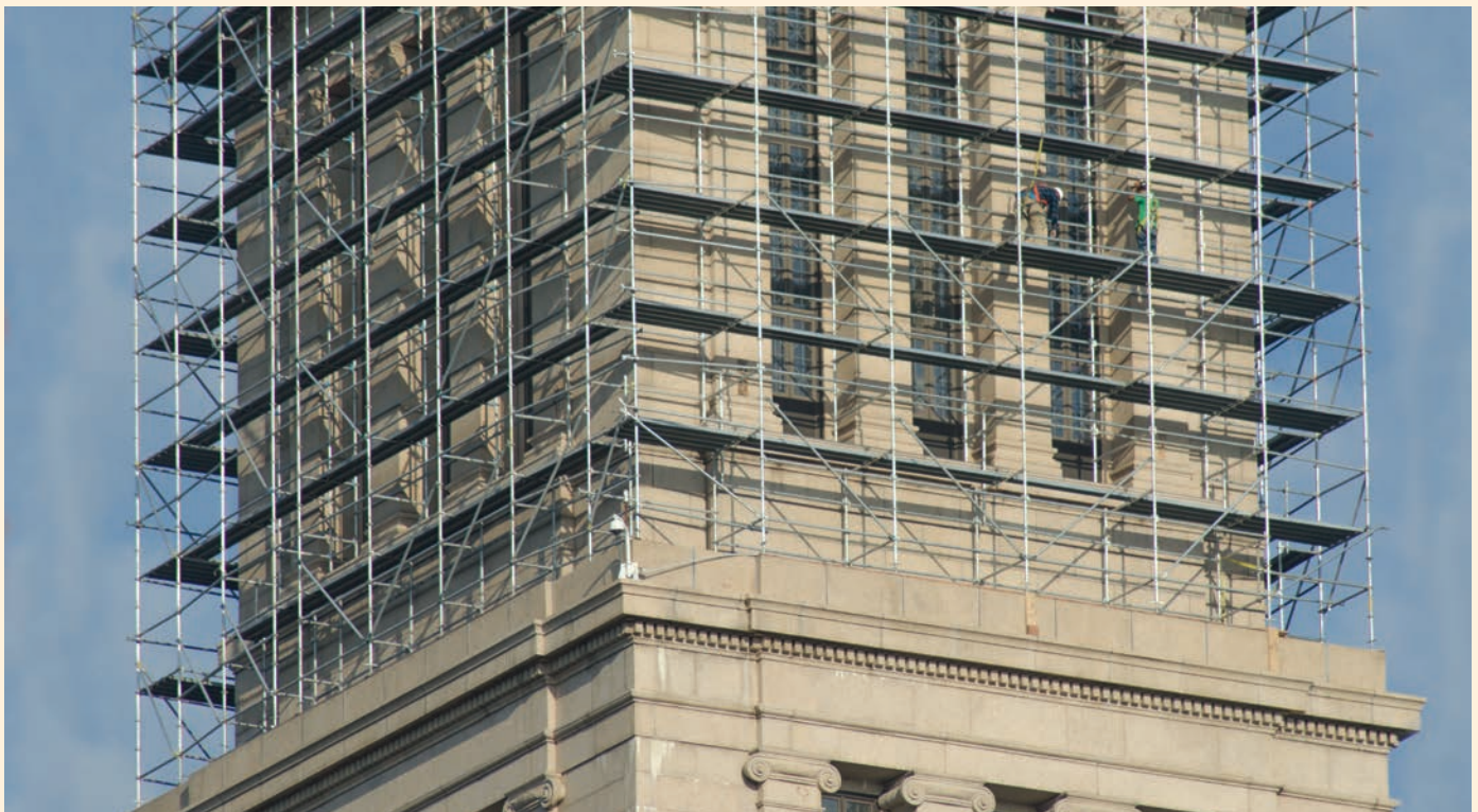
High on a scaffold on the eastern face of the Eighth Floor (Templar Chapel), workers carefully remortar the Corinthian pilasters.
